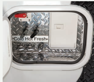
Plumbing Control Panel
